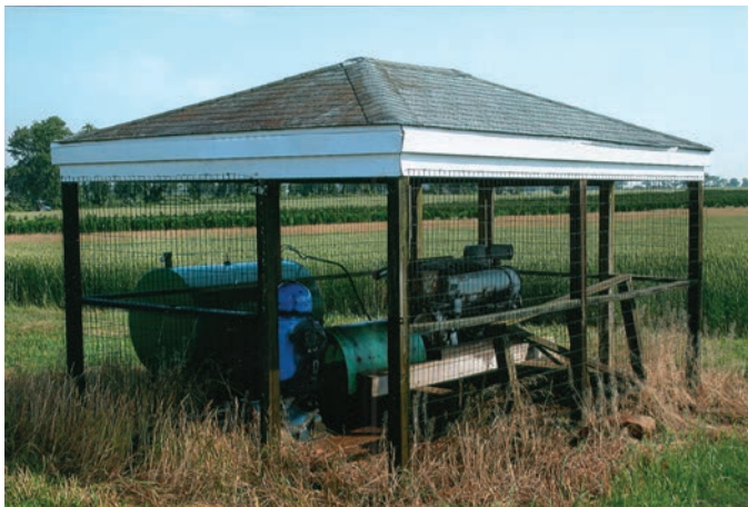
The pump house with its open wire mesh around the outside allowing birds to fly through or use the walk-in entrance. Naturally the parents chose to use the entrance!
